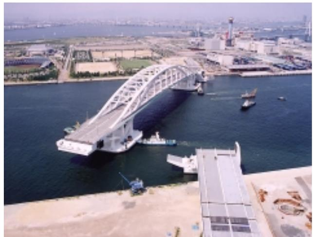
Photo 12 Floating Bridge Is Being Installed at the Site
