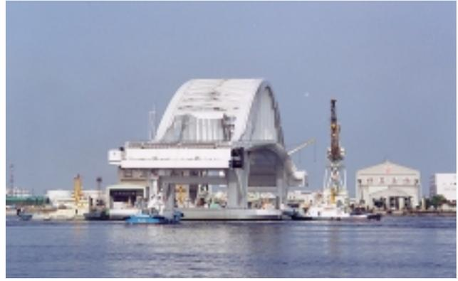
Photo 10 Floating Bridge Is Being Pulled out of the Dock
