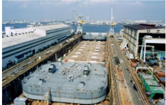
Photo 6 Pontoons Installed
